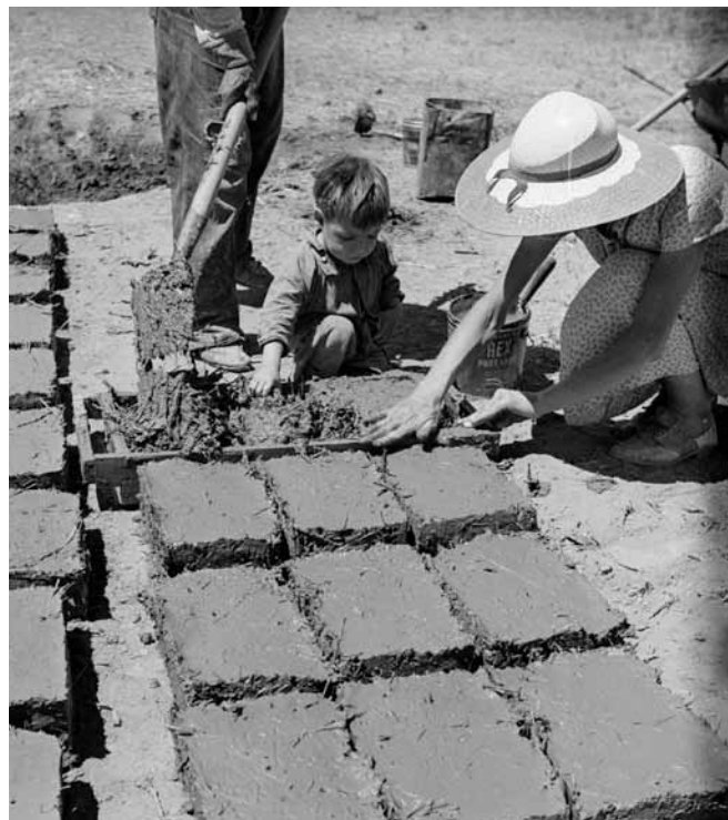
Above left - Water was essential for house construction. Here we see Ricardo Archuleta mixing mud to make adobes. Behind him are Patricio, Clarence, Alicia, and Juan Archuleta. Above center - Juan and Alicia smoothing the mud in the form before Ricardo lifts it off. Above right - Water was also important for public works, here community members making bricks to build the Ranchos public school, a WPA project. On the left is possibly Juan Dolres Gonzales, in back is Andres Maestas, and on the right is one of the Valerios - Leandro, Eduardo, or Ben. Note the bank of the then newly enlarged Talpa deposito in background. All photographs 1939 or 1940.
